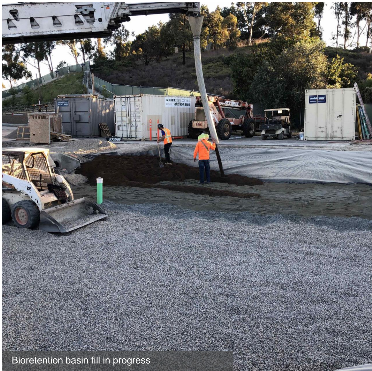
Bioretention basin fill in progress
