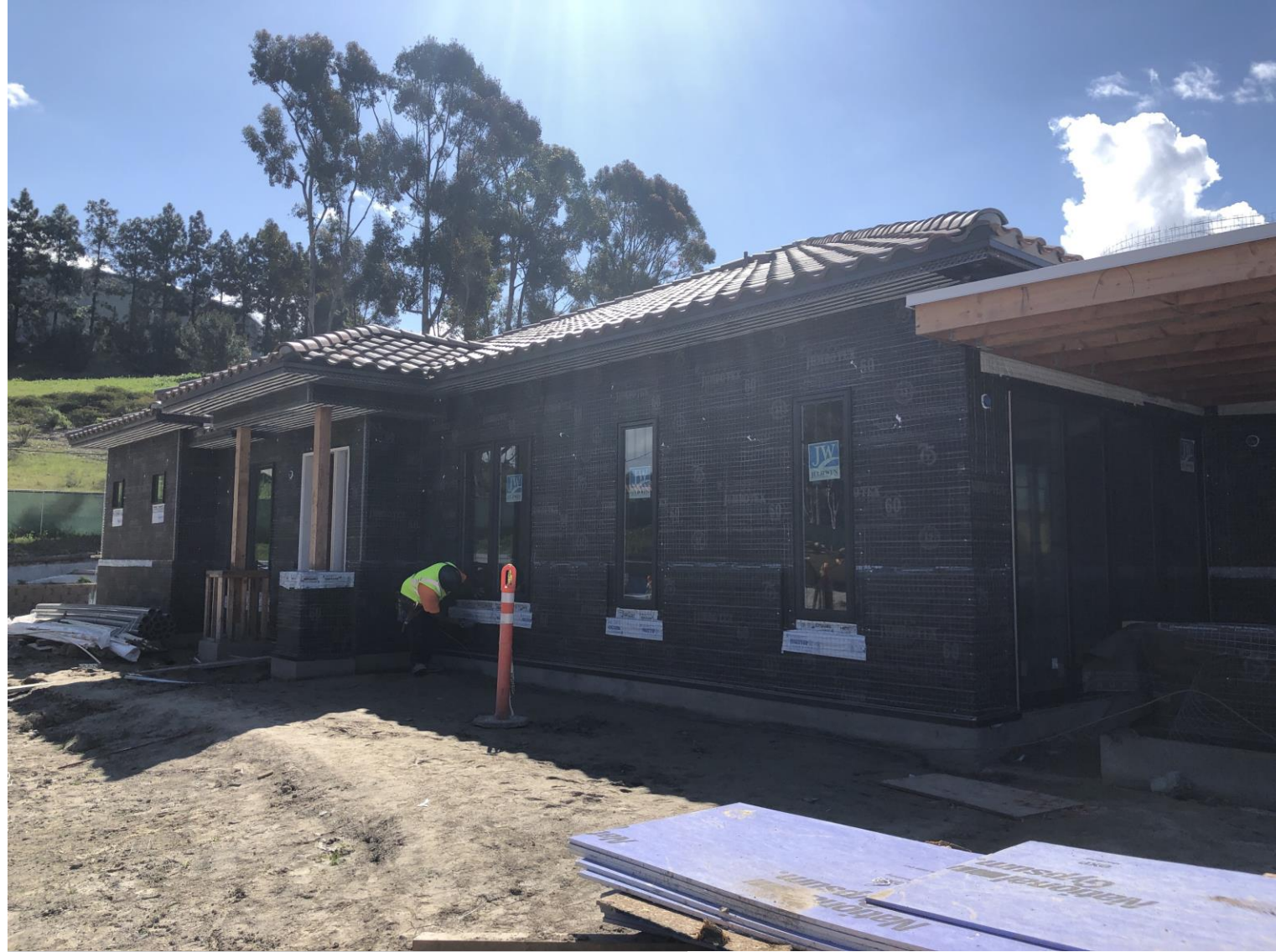
Cottage exterior window and lath install
