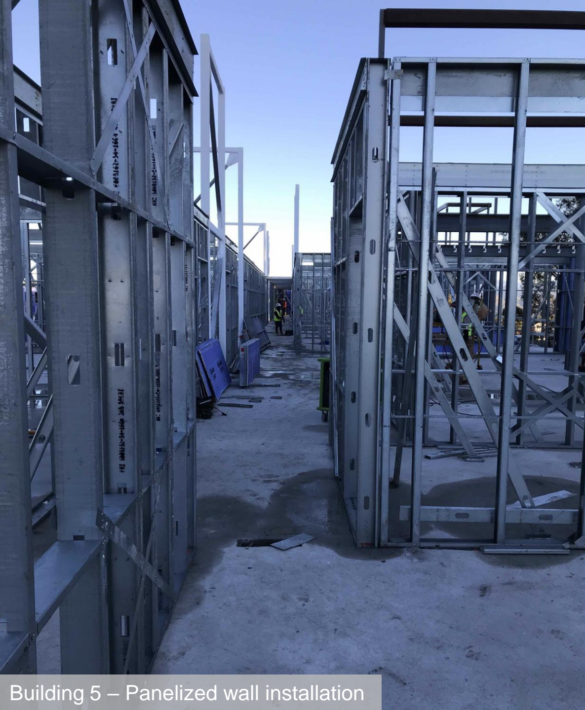
Building 5 – Panelized wall installation
