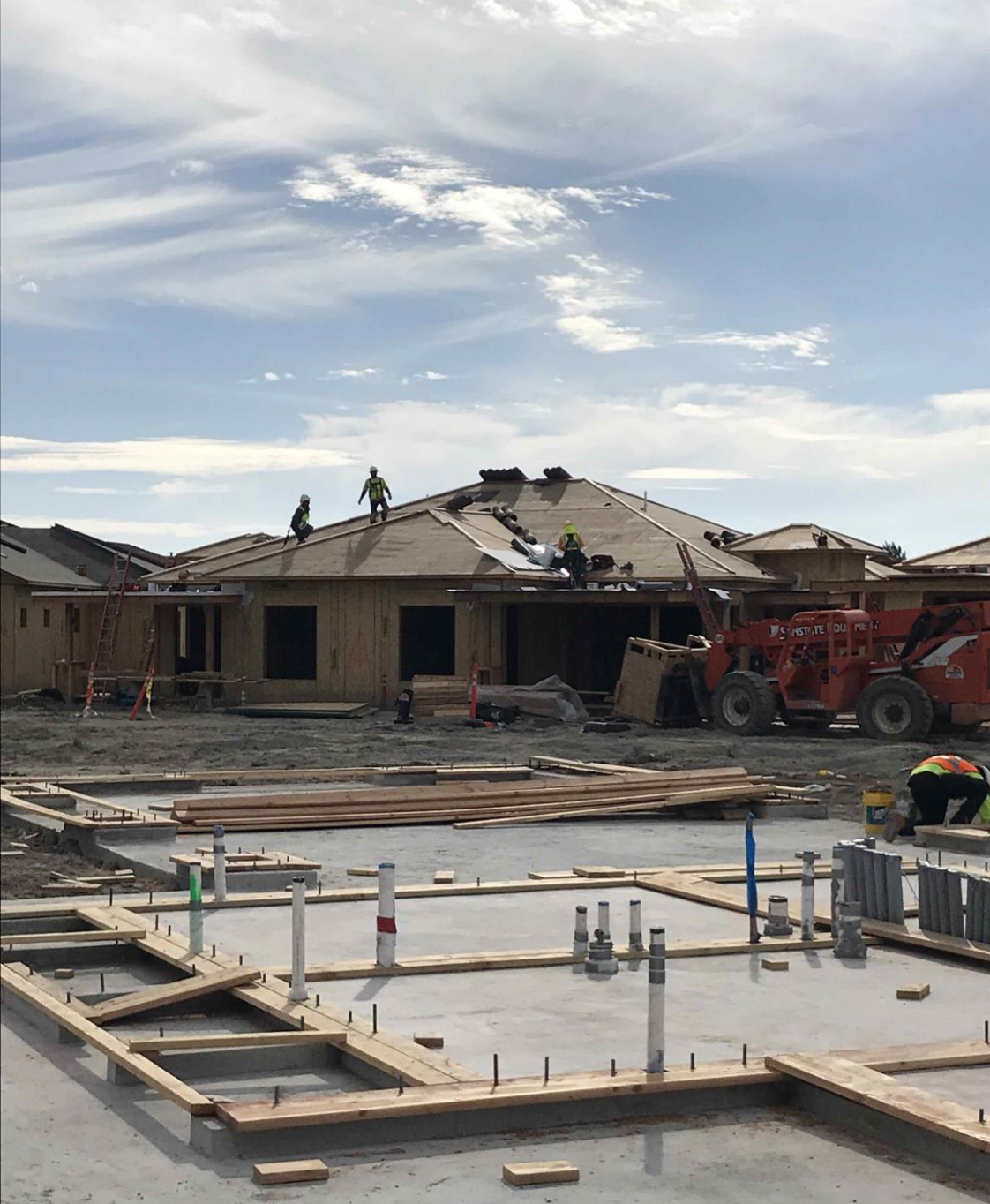
Building 10 layout, SW Cottages roofing dry-in
