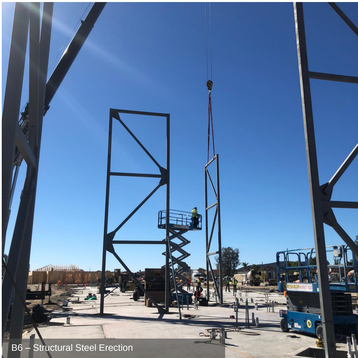
B6 – Structural Steel Erection
