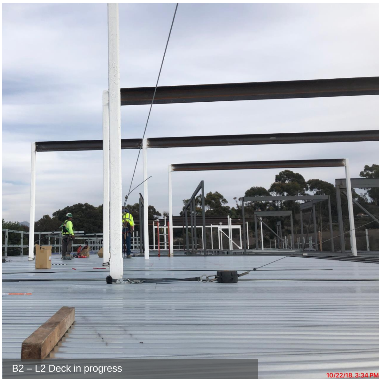
B2 – Joist Framing/L2 Deck in progress
