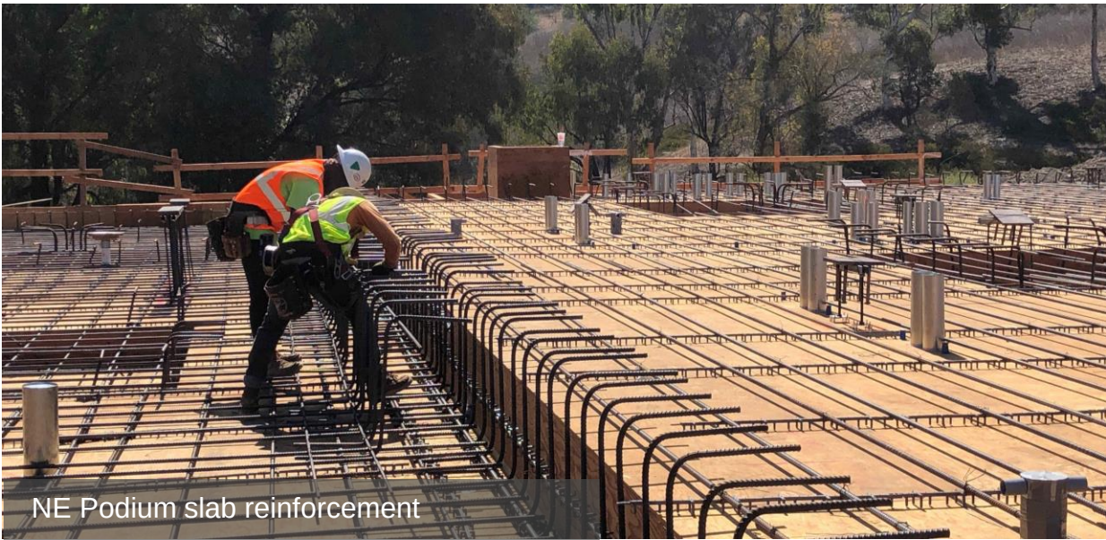
NE Podium slab reinforcement
