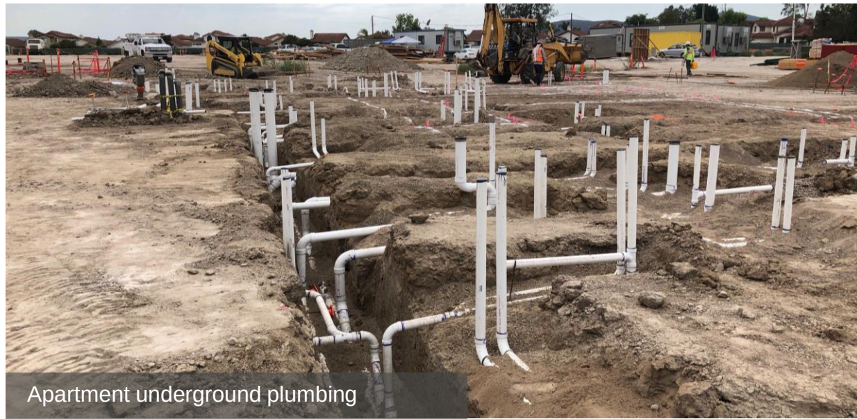
Apartment underground plumbing
