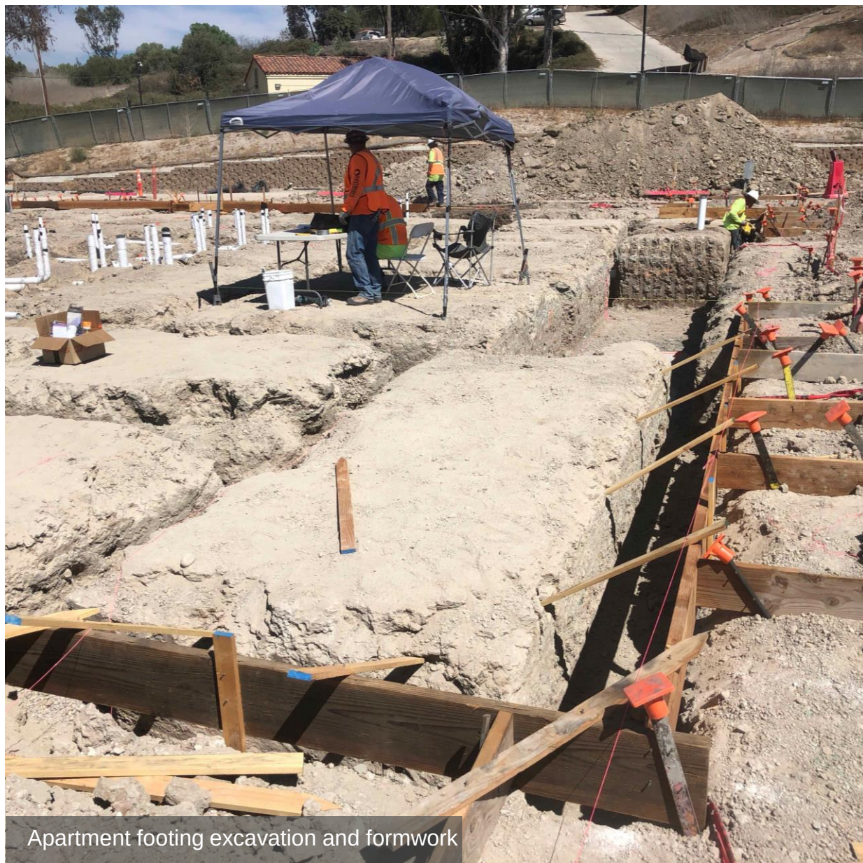
Apartment footing excavation
