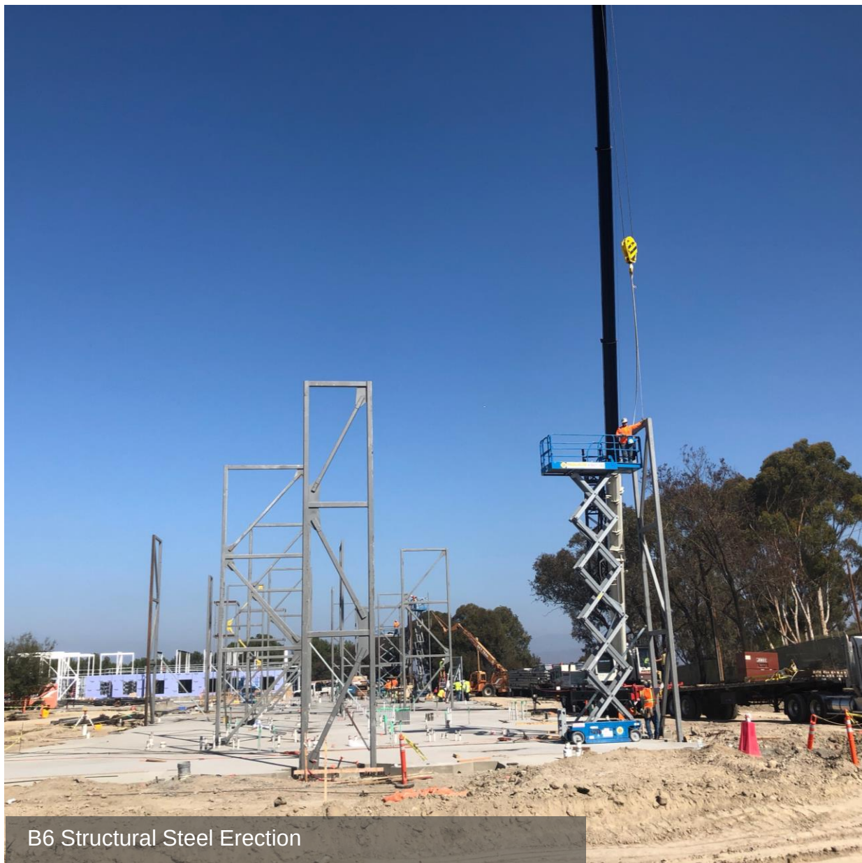
B6 Structural Steel Erection
