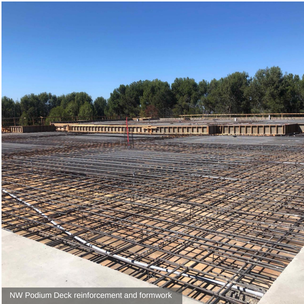
NW Podium Deck reinforcement and formwork
