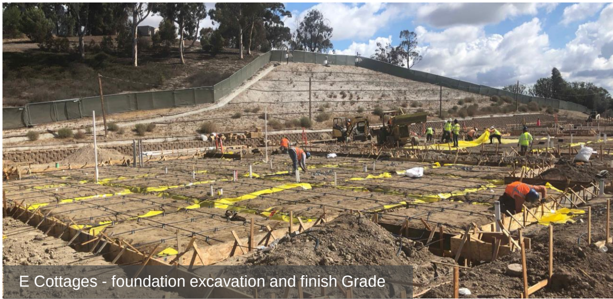
E cottages - foundation excavation
