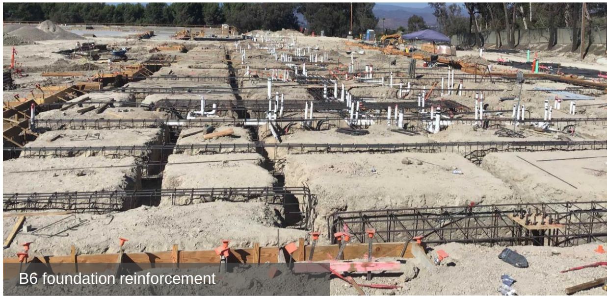
B6 foundation reinforcement
